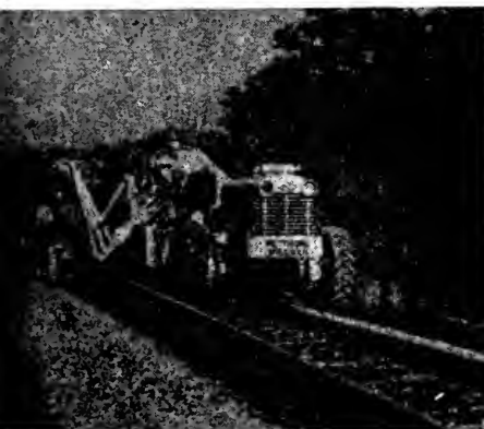
LAYING WELDED RAIL
